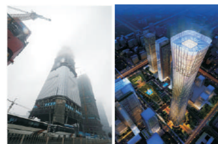
The control system for the Die Climbing Machine ,which used to build the China Zun , the tallest skyscraper, is designed by our company .
